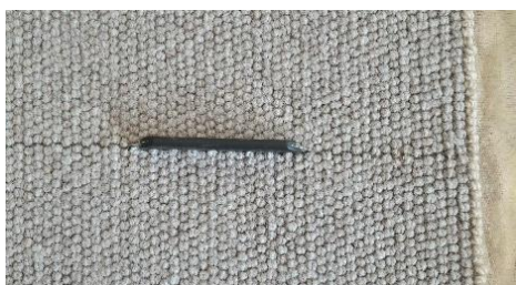
Photo 3: Use a fine bladed row finder to open the pile across the carpet.
