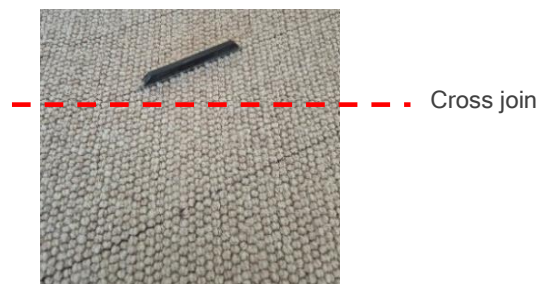
Photo 4: A fine bladed row finder through the angle will assist lining up the cross join.
