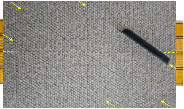
Check the join aligns through the angle
